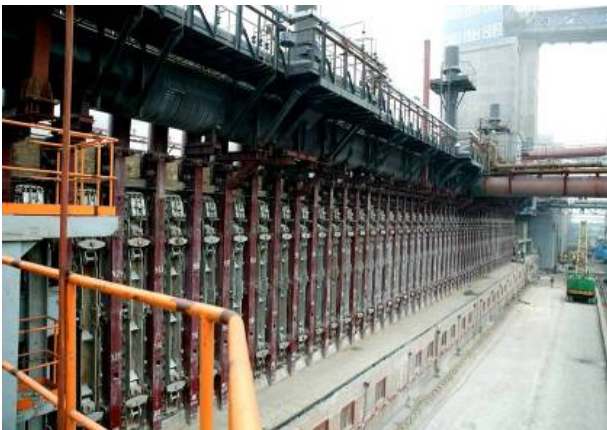
Figure 1. Coke furnace battery No. 4 of coke department No. 1
