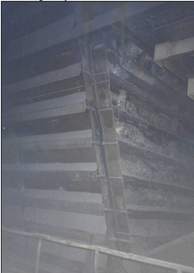
Figure 2. Repaired bearing stiffeners of the hoppers
