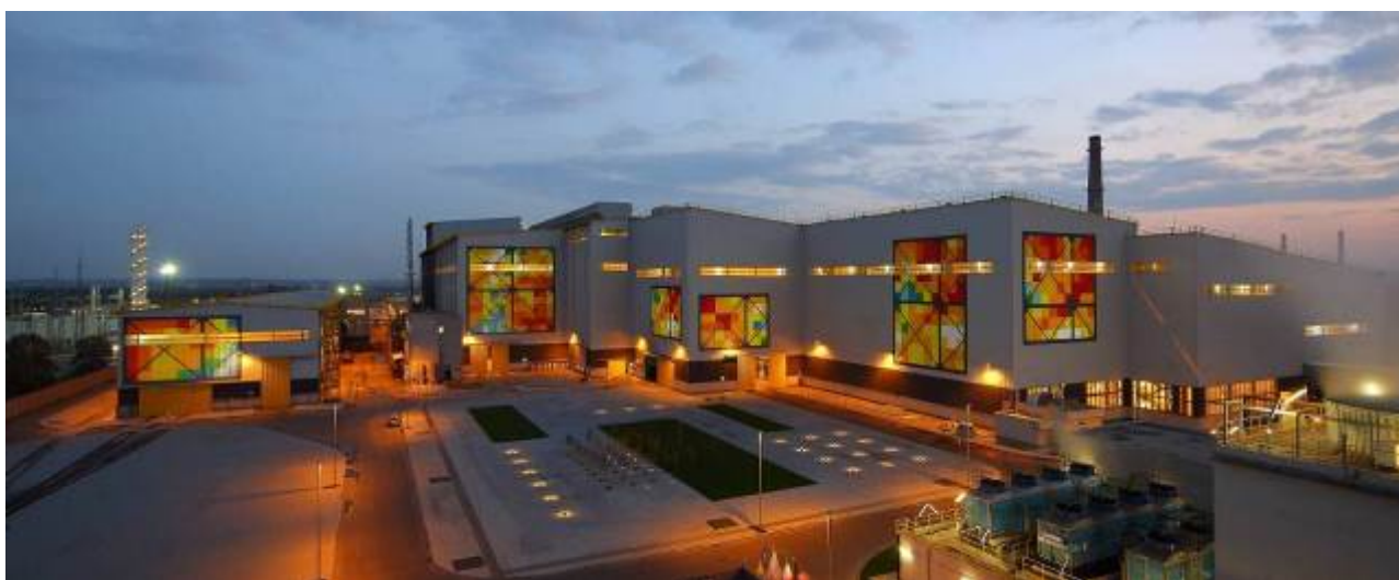
Figure 2. Interpipe melt shop front view
