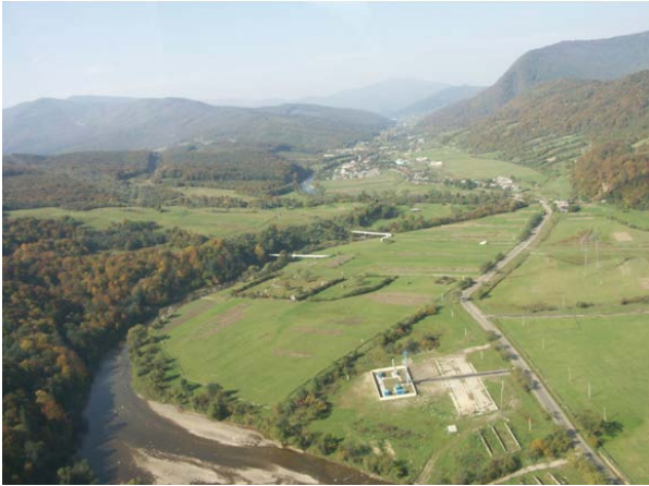
Figure 2. Aerial crossing of MP “Urengoy-Pomary- Uzhgorod” through the river of Limnitsa
