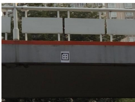
Figure 9. The Position of Target Marker in Test Bridge
