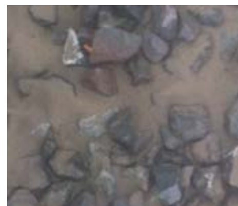
Figure 2 (a). fine sand with ballast (40% fouling)
