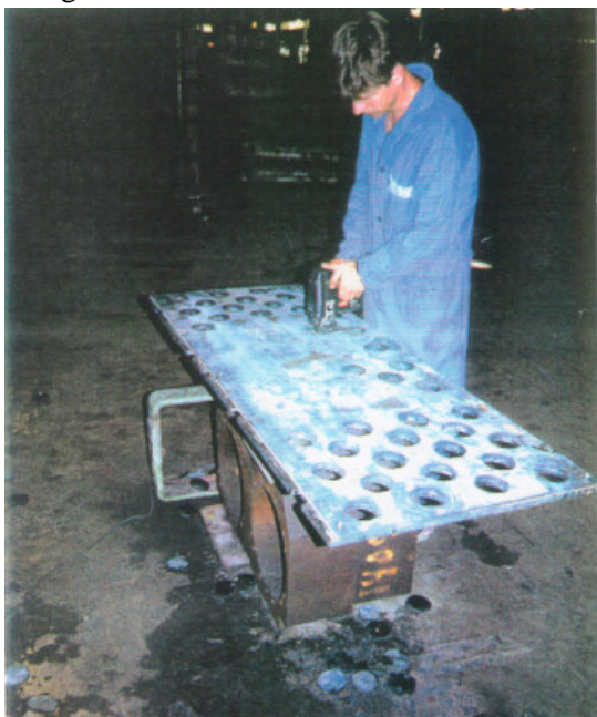
Figure 3 Reconstruction of screen deck surface
